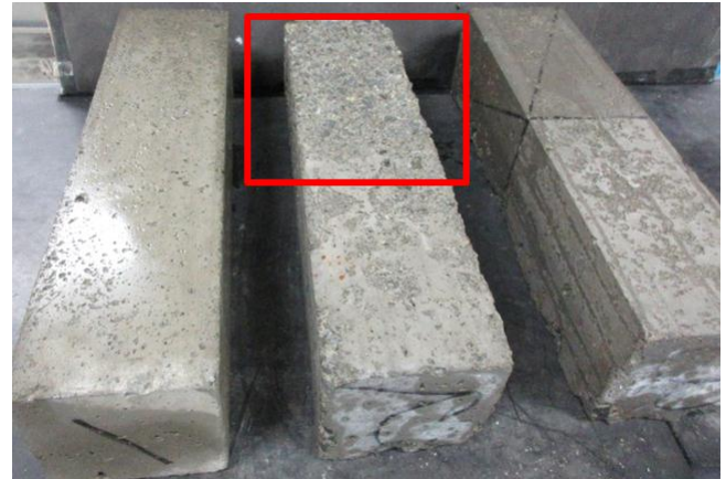
Figure 9 Initial peeling damage of the coating area by surface impregnation materials
